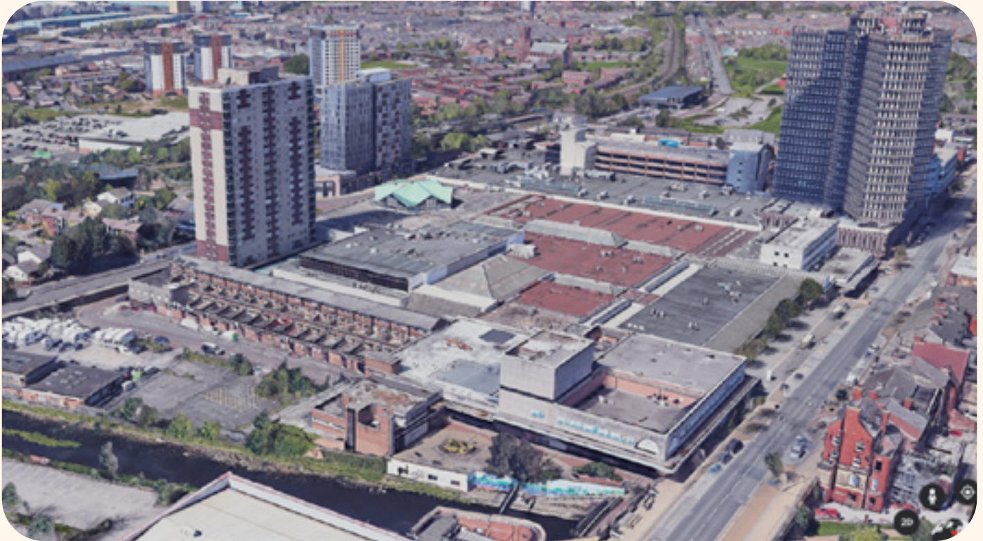
Figure 7. Strand Shopping Centre, viewed from the south towards Seaforth
