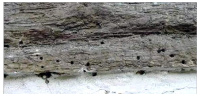
Round and dark holes indicate historic beetle attacks, whereas active infestations have sharper and lighter holes
