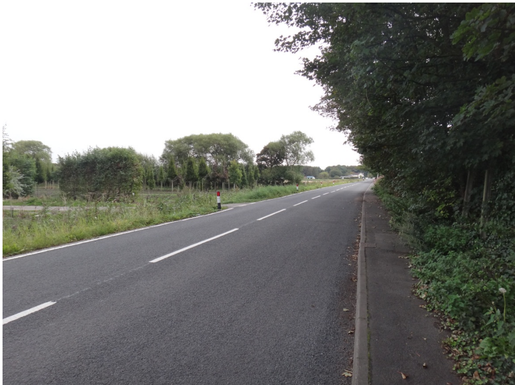
Figure 3: Narrow Footway at Site Access
