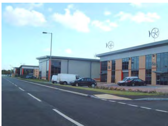
New business units at Bridle Road Industrial Estate
