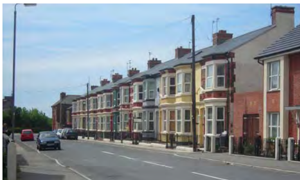
Refurbished terraced housing in Bedford Queens Housing Market Renewal area, Bootle
