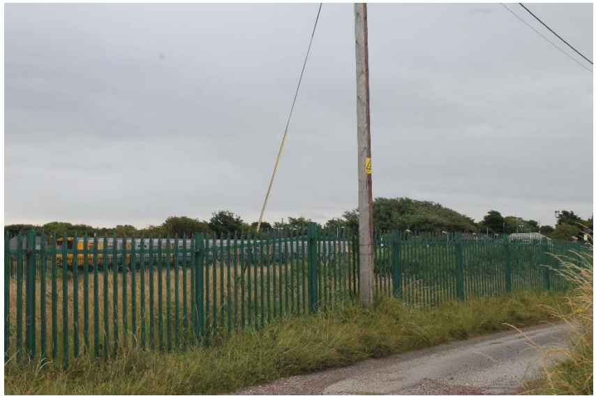
VP2. View looking east across site from western boundary of site
