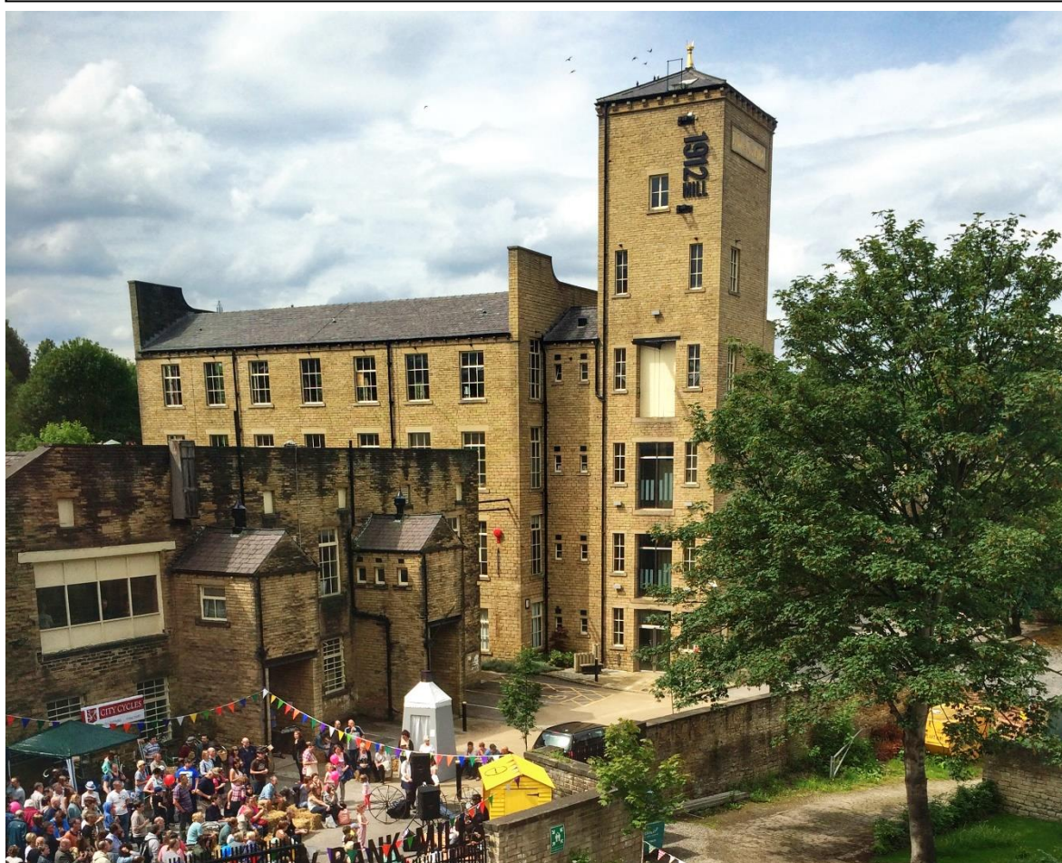
2 Sunny Bank Mills, Farsley, Leeds
