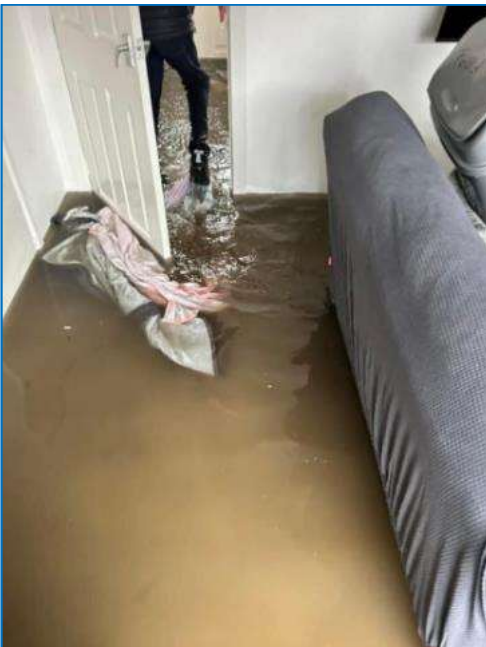
Figure 7: Internal flooding on Bulwer Street 30 th September 2024
