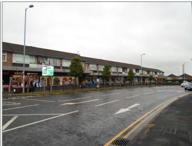
Shopping terrace, north side of Westway.
