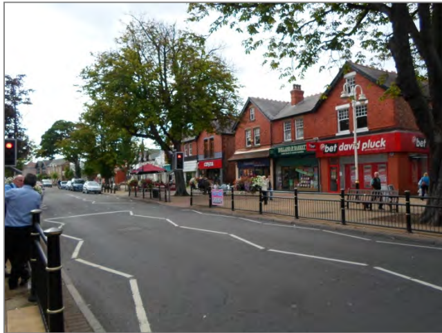
Retail units on Chapel Lane.
