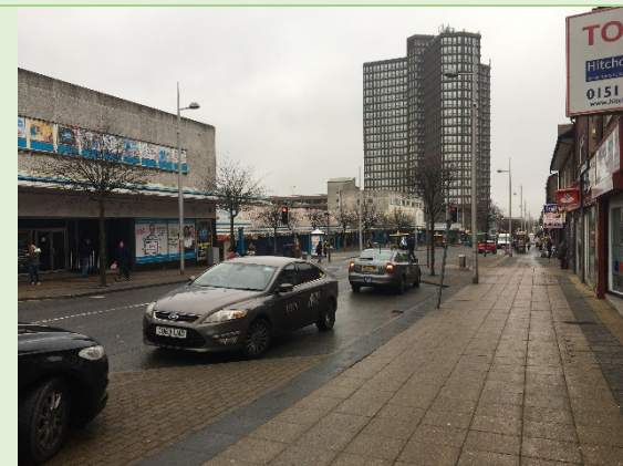
Figure 4: View towards The Strand Shopping Centre from retail units on Stanley Road
