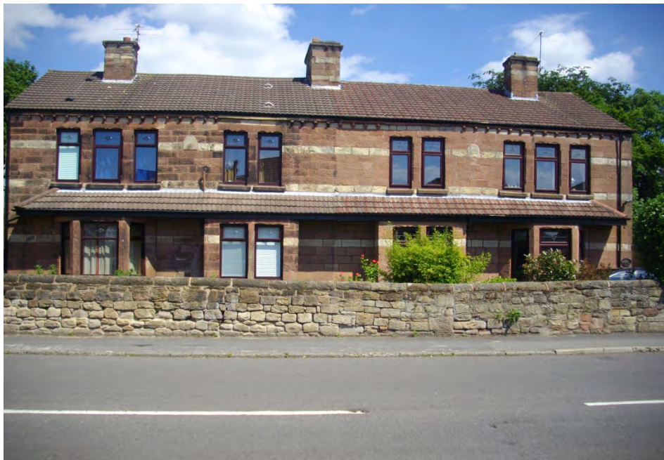
158 – 160 Liverpool Road South
