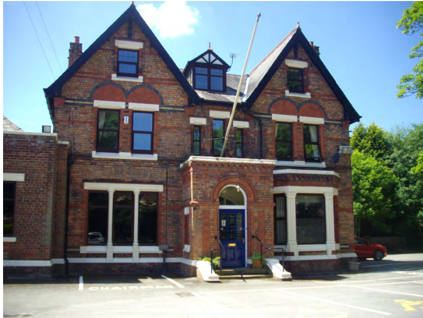
Kensington House, Station Road
